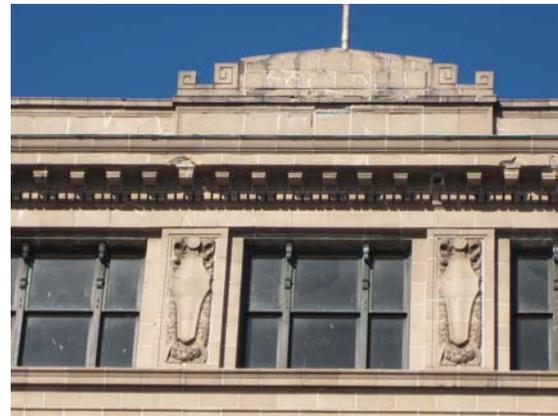
the northwest corner of the Union and State Streets intersection). The gable at the top of the building façade, pictured here, was removed, and netting was wrapped over the front of the dental molding and cornice to prevent pieces of the façade from falling to the sidewalk below.
