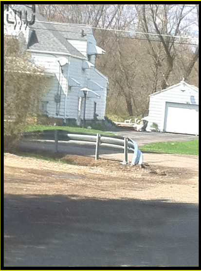
Cattaraugus County replaced a guard rail on Delaware Ave.
